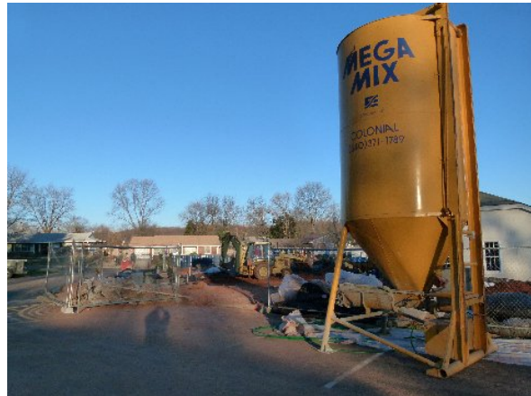
Mortar mixer for new walls, the week of January 3, 2011
