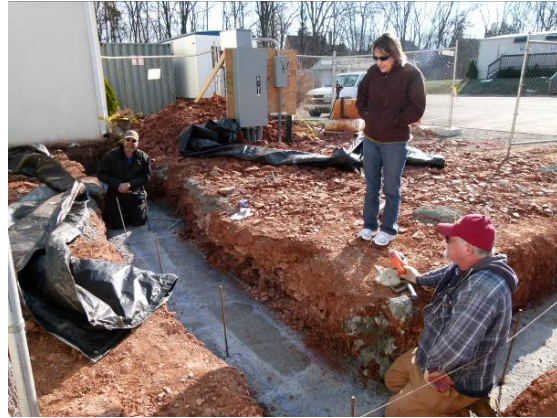
Working on the footings, December 2010
