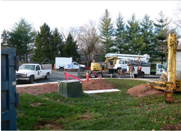
Relocating the transformer, December 2010
