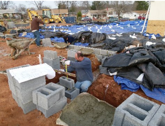
Sully Construction working on New Year's Day
