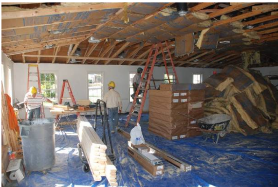
Reinforcing Roof Trusses, November 2010
