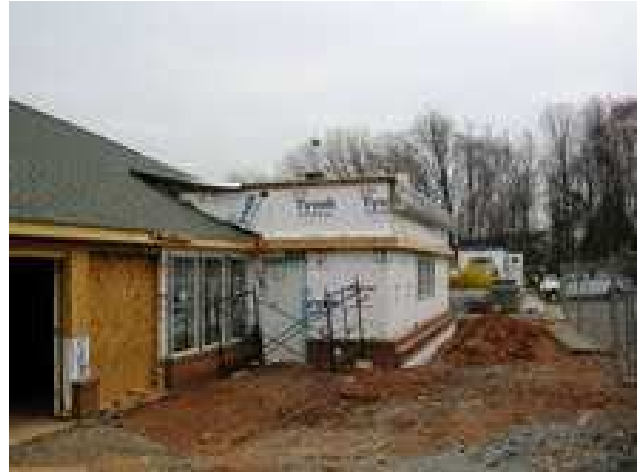
Kitchen Roof Construction
